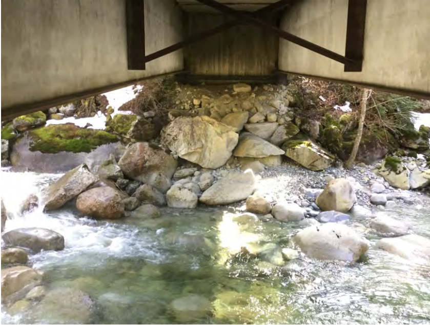
Left Bank Abutment when facing downstream
