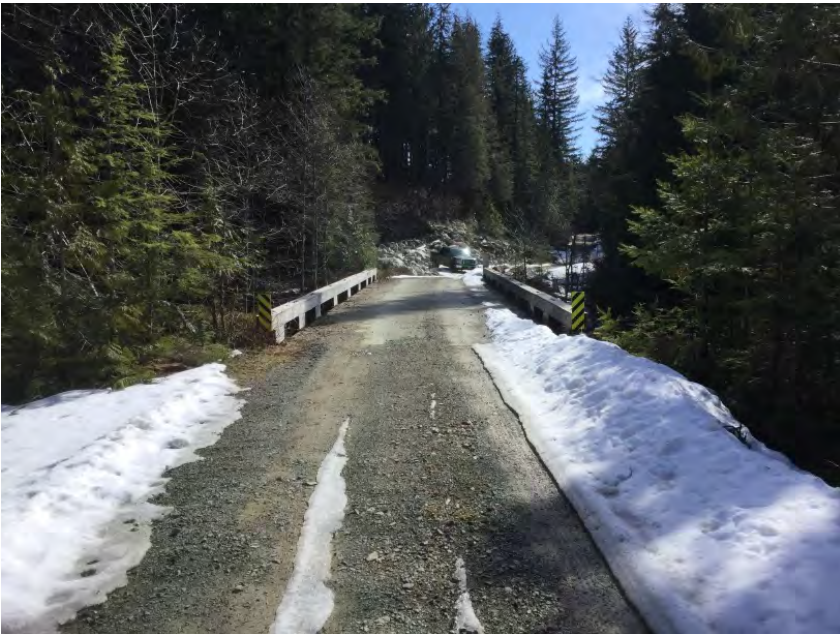
Approach from Right Bank when facing downstream
