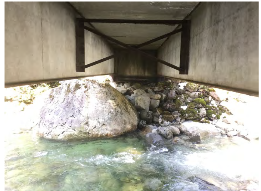
Right Bank Abutment when facing downstream
